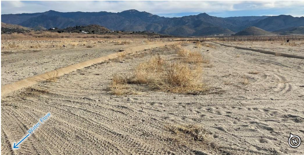
**Figure 2-9. Canal Filled with Sedimentation, Looking Upstream (Downstream of Tilley No. 2 Concrete Flume) (Photo Date: 03/2022)**
