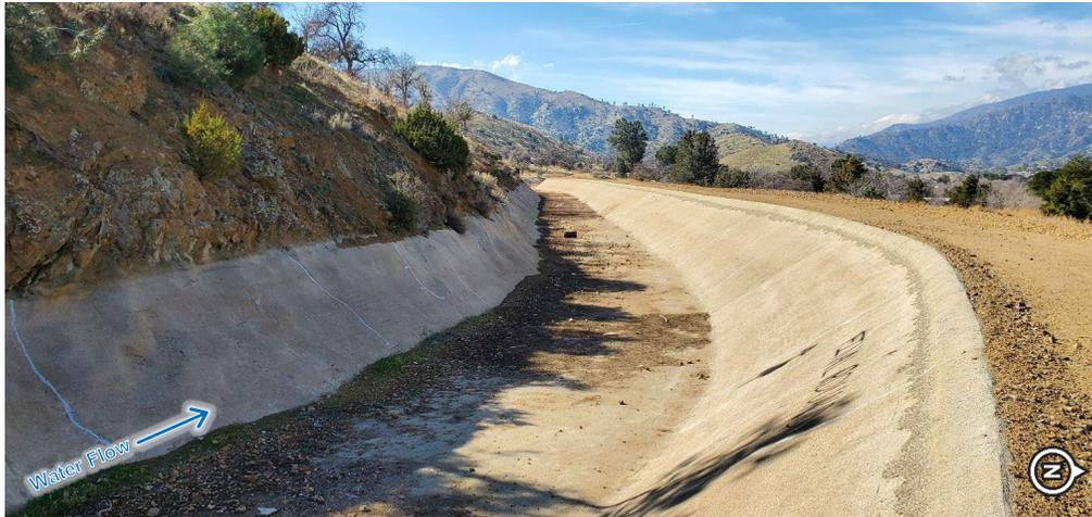
Figure 2-39. Concrete-lined Canal, Looking Downstream (Photo Date: 01/2020)
